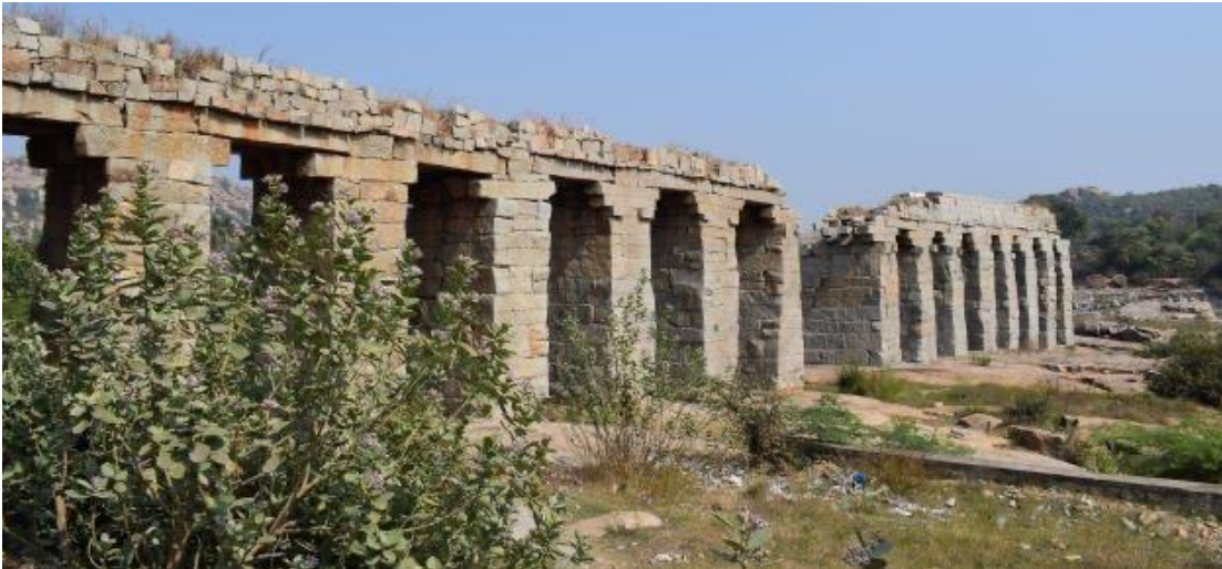
Fig. 33: Bukka aqueduct, Hampi, Karnataka
