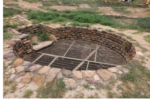
Fig. 7: Rock-cut reservoir inside East Reservoir
