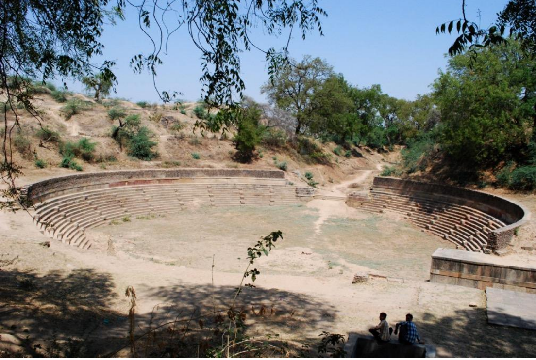
Fig. 26: Circular desilting tank, Sahasralinga talav, Pathan
